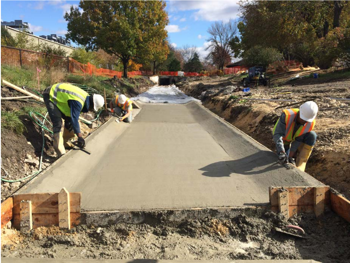
(Middle) 1500' Concrete Water Diversion Canal Green Field Site Madison WI 2015
