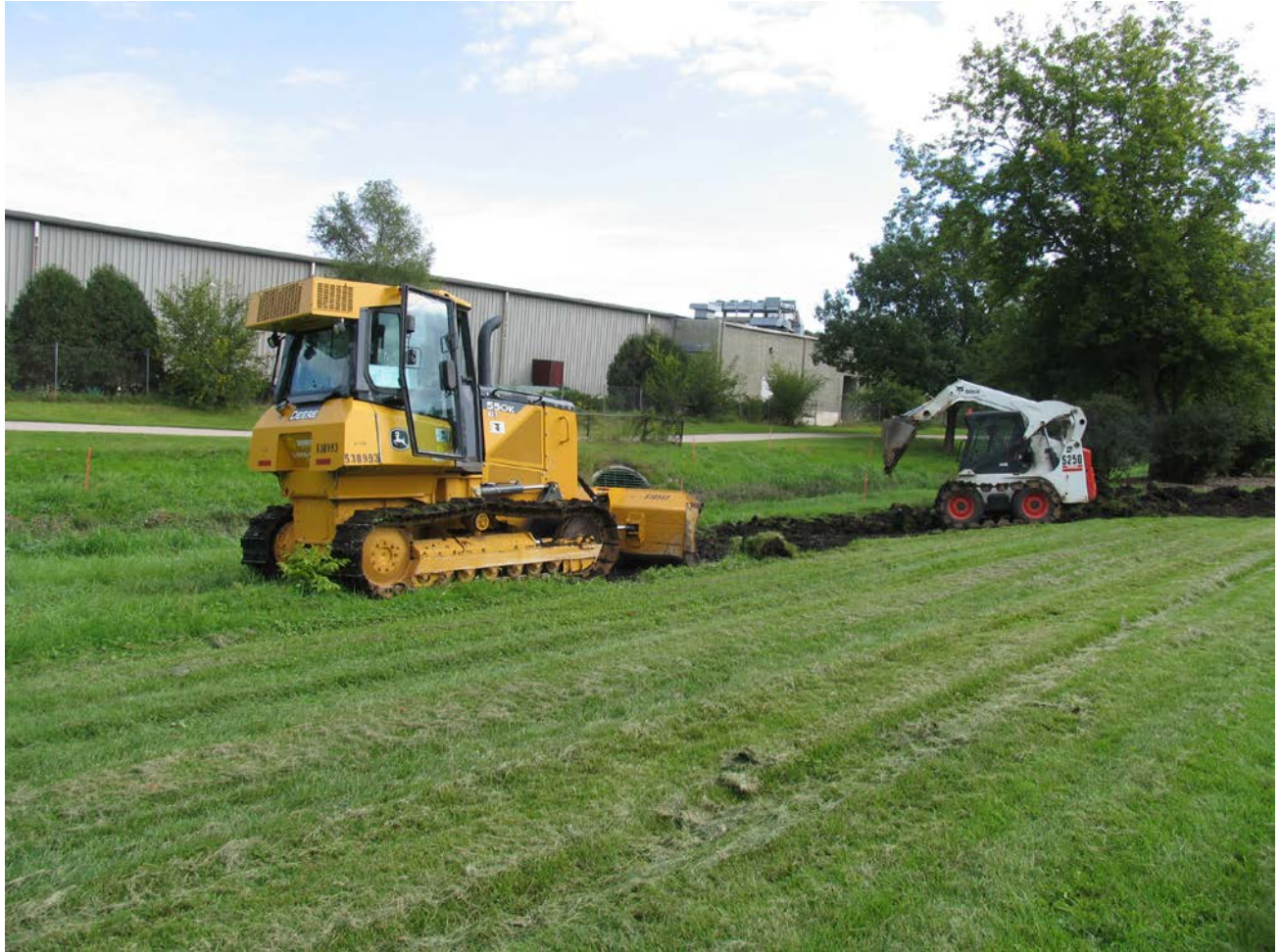
(BEFORE) 1500' Concrete Water Diversion Canal Green Field Site Madison WI 2015
