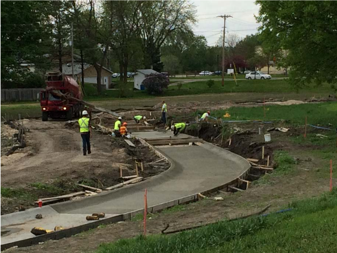
(Near End) 1500' Concrete Water Diversion Canal Green Field Site Madison WI 2015
